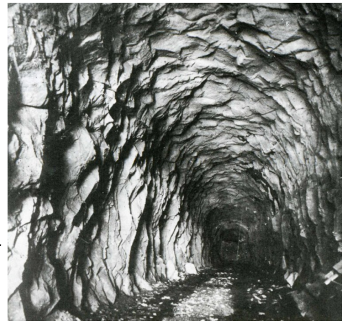
Chinese drilled and blasted a 1,659 foot tunnel through the Sierra Nevada for the C.P. Completed in 1867
