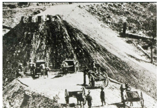
Using picks and shovels, carts, one-horse scrapers, and black powder graders about 20 miles of bed at a time, blasting hills and filing large ravines.
