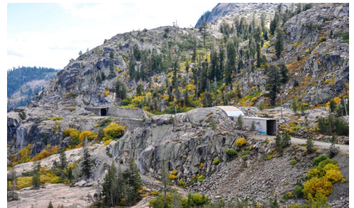
Transcontinental Railroad track #1, Donner Summit Tunnel #6 (1,659 feet long-same as above). First use of nitro glycerin blasting. Two years in construction. Opened in 1867, now abandoned.
