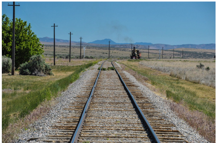
Looking along the original 1869 grade as the U.P. locomotive 119 approaches Promontory Summit. The tracks are new, but the grade is the same as on May 10, 1869. This section is the last 2,500 feet of the Union Pacific Railroad before connecting with the Central Pacific at Promontory Summit on May 10, 1869. The view is towards the east.
