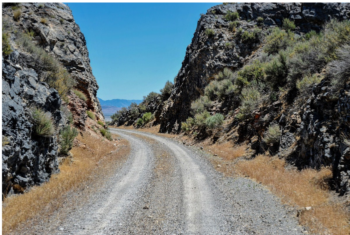
The last cut made by the Union Pacific on May 6, 1889. You can still see the marks made by the blaster's drills as they drilled the hole to place the black powder for blasting out the rock. This view is to the southeast and the Great Salt Lake Basin. The grade is approximately 15 feet wide through this curved cut.
