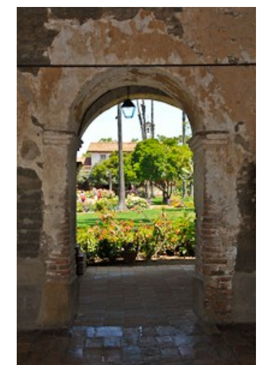
Looking into the Main Patio
